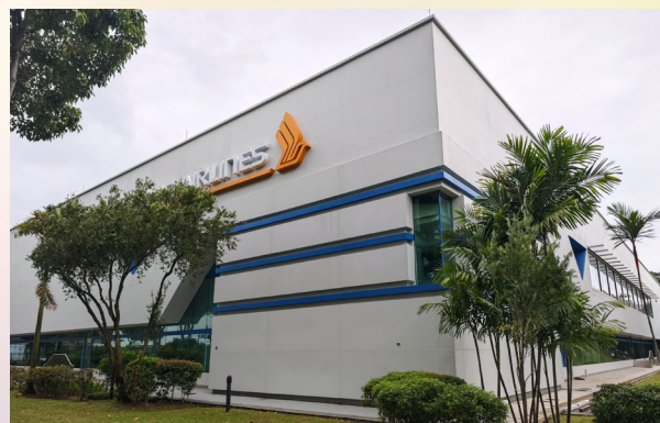
SBO facade with cool paint
